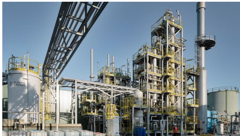
Figure 18: Plastics Energy Chemical recycling facility in Spain at an industrial scale
